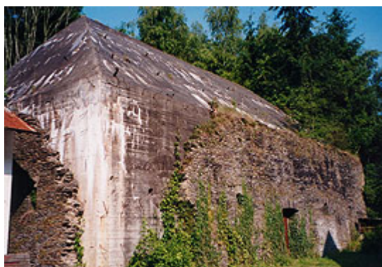
Adlerhorst: Guardhouse bunker. Note the facing. Some wood and paint, and it would look like any house.
